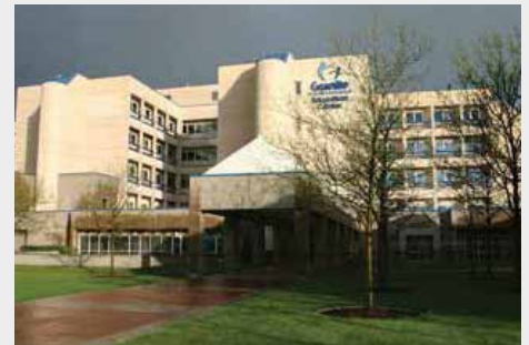
Granite School District's administration building also houses the Granite Technical Institute and leases some space to Utah State University, requiring 24/7 access that increase the need for access control.
