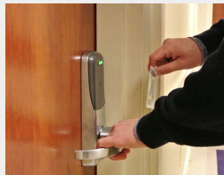
The university integrated Scchlage AD Series wireless locks with BadgePass TotalCard to better control access rights in residence halls.
