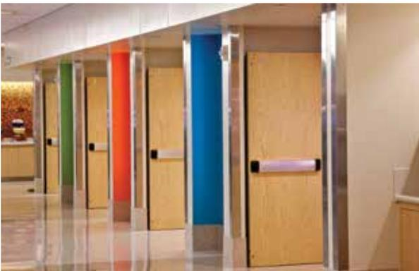
Stainless steel—a steel alloy mixed with chromium—does not readily corrode, rust, stain or show fingerprints. However, its shiny appearance doesn’t always fit with the design look of the building. Satin stainless steel or satin chrome are often chosen as alternatives.
