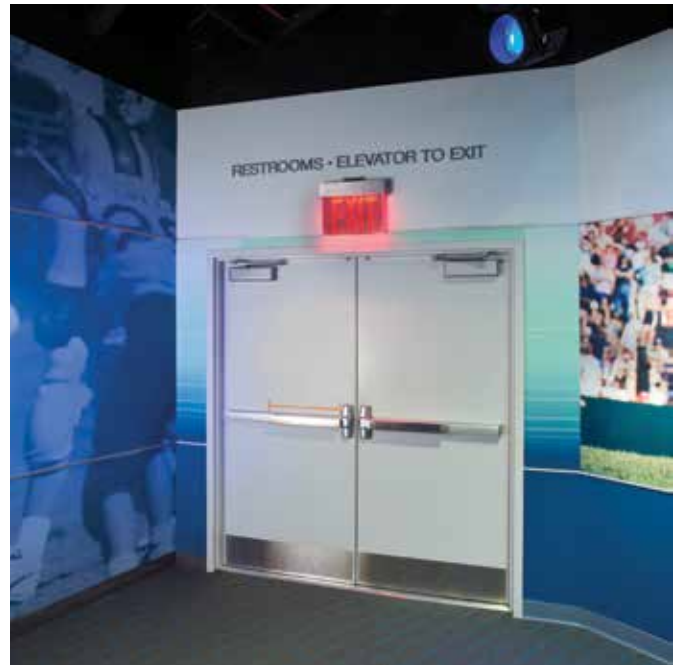
The actuating portion of panic hardware must measure at least half of the door width.
