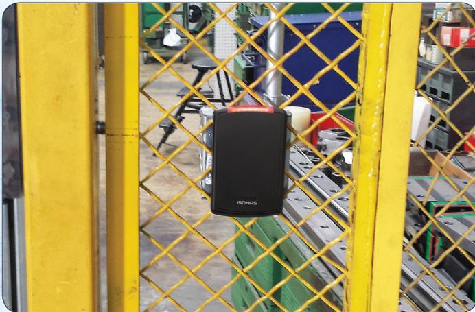
The ISONAS RC-04 reader controllers were installed on the secure gated cage within a day of the project being approved, beating the audit deadline. The additional reader controllers were installed on the remaining doors as the locksmith completed installation of lock mechanisms and repair of problematic doors. With all the pieces in place, NHG was able to work together with ISONAS to provide a state-of-the-art access control solution in no time, creating a win-win situation for all.
