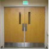
Helpful Hint: Limit the entry points to as few as possible and use door position switches to monitor opening and closing.
