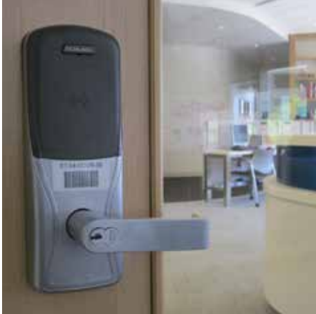
AD-Series locks were added to openings that separate public areas from restricted areas, such as private offices or cross corridors between buildings.
